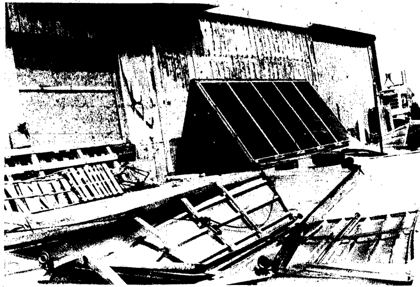
BOARDED UP entry ways and charred siding are mute reminders of a fire Wednesday at the Laurel Ready Mix plant in which plant owner Leon May received serious
